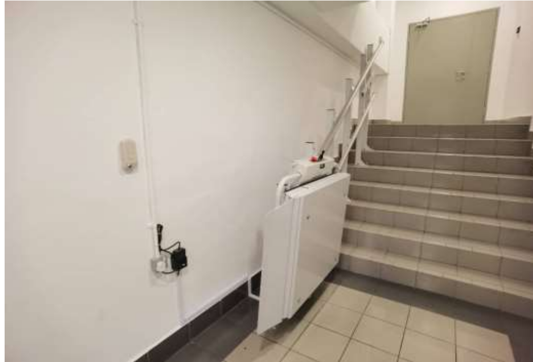
Installation of OKU Stairlift Platform Menara Axis
